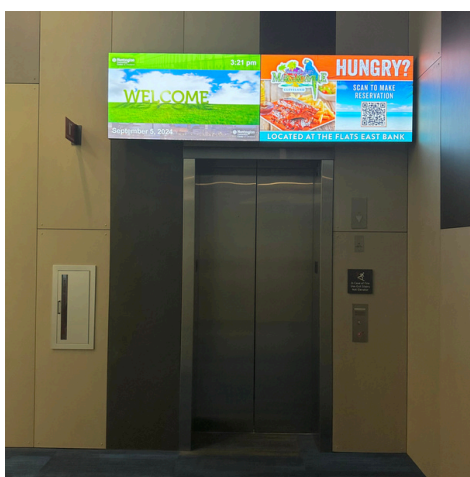
Exhibit Hall Level Elevators
