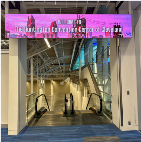
Hall A - Upstairs
