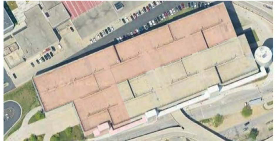
Remaining Structure Demolished
