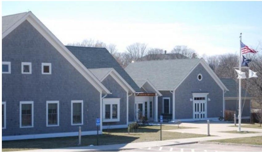
Figure 27. New Shoreham Town Hall (Turaj, 2013).
