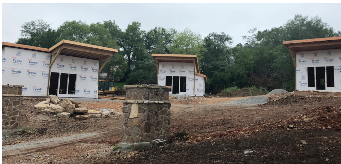
Figure 4.6: Tiny homes under construction
