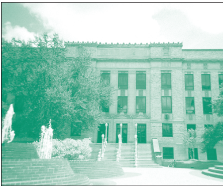
Chemistry Building (Texas A&M University)
