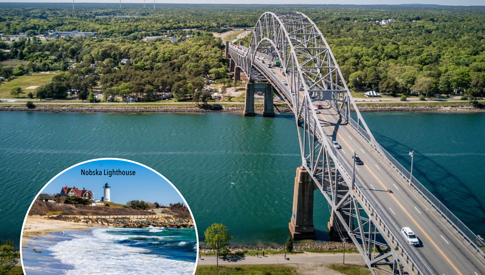
Bourne Bridge on Cape Cod Canal
