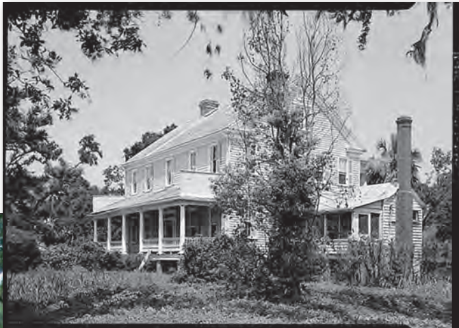
(Left) 1990 HABS Photograph of the McLeod Plantation House.
