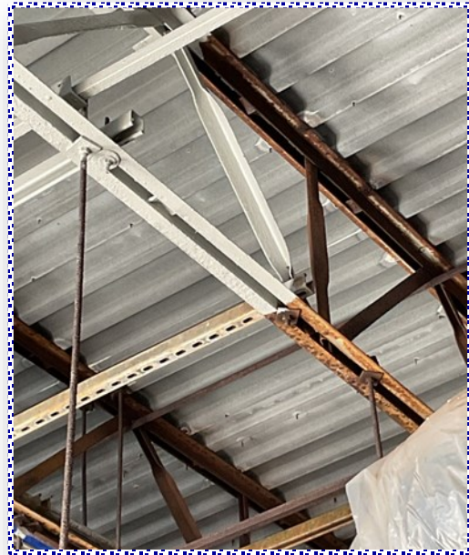
New primer and white paint on roof deck and trusses
