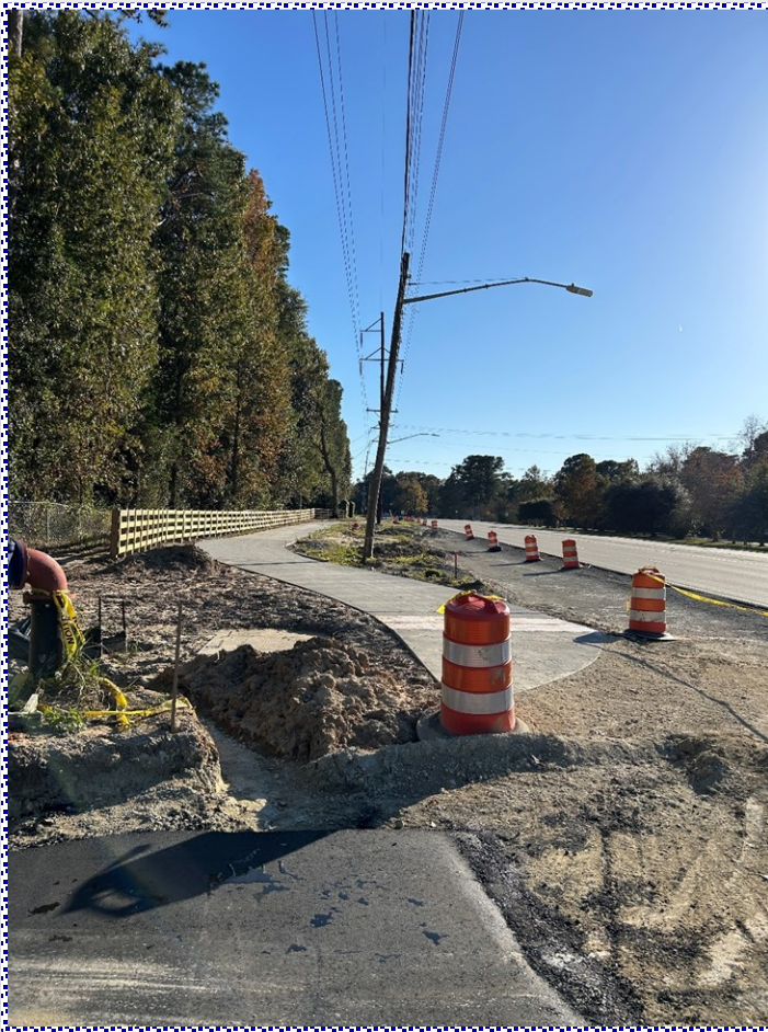
Turning lane graded and ready for asphalt
