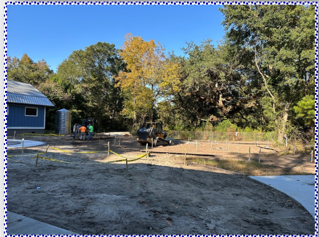
Top: Entrance road asphalt paving Bottom: Rain Garden paths grading
