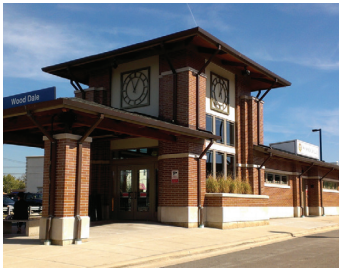
Wood Dale Metra Train Station
