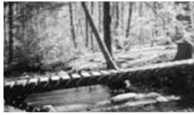
Bridge across Toms Run.
