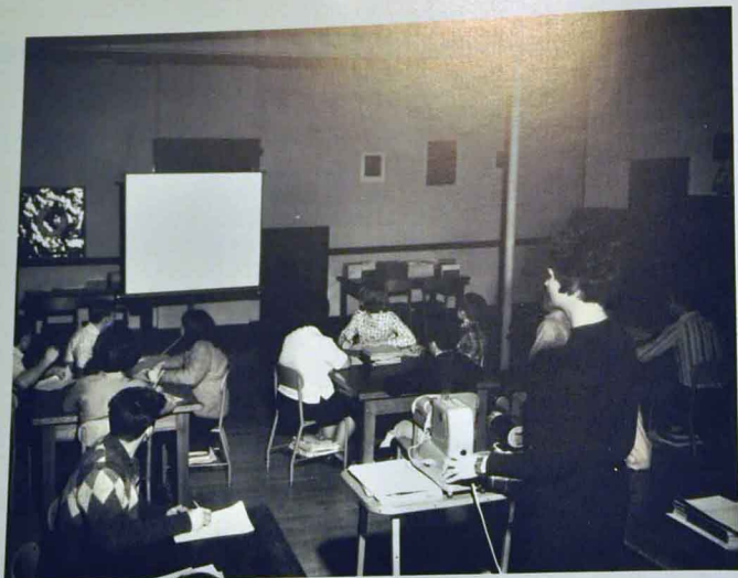
Mrs. Marilyn Brown, reading improvement instructor, captures the attention of a freshman class with the Tachistoscope. This machine, flashing numbers on a screen at a timed rate, increases visual acuity of students.
