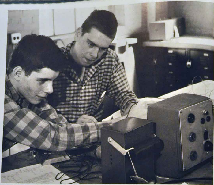
Students in Mr. Davis' electronics class use the vacuum tube volt meter to run tests on equipment.
