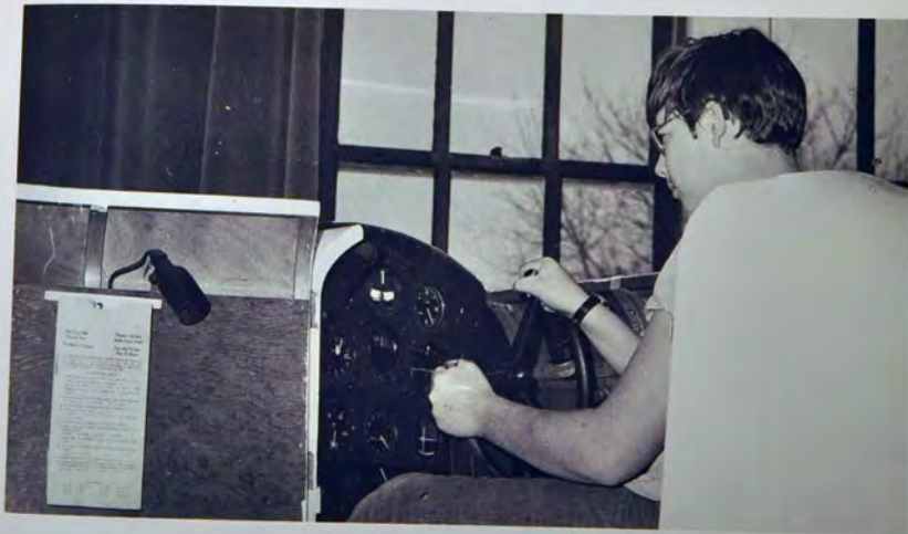
Aviation science students experience the sensation of actual flight in the Link trainer, which is fully-equipped to simulate all the aspects of flying.
