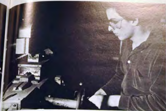
Surface grinders smooth and even out rough edges on Ken Levey's project, a drill press vice. Ken chose to construct the vice to have the benefit of its use on future projects.
