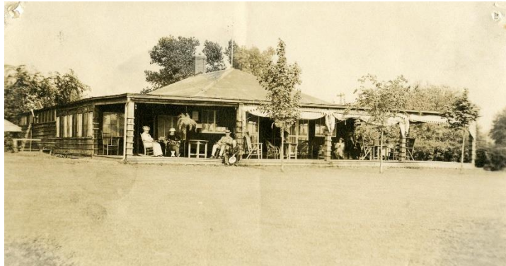
Elmhurst Golf Clubhouse, designed by Walter Burley Griffin. M88.15.13
