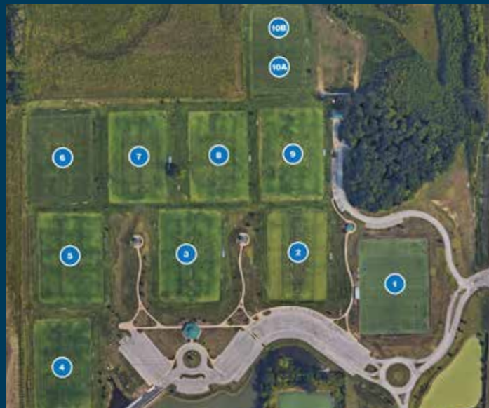
Goebel Sports Park consists of 10 full-size fields—two synthetic turf, six bermuda grass, and two cool season grass. Six fields have lights. A training room and concessions are also available.
