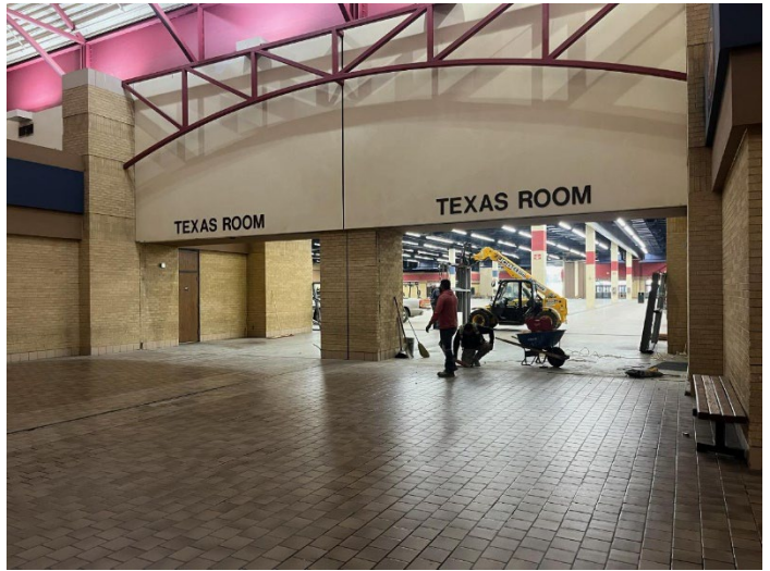
Replacement of Exhibit Hall doors.
