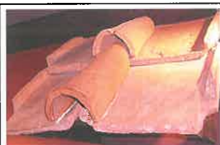
An example of how tegulae and imbrices created a typical Roman roof (© Fishbourne Roman Palace)
