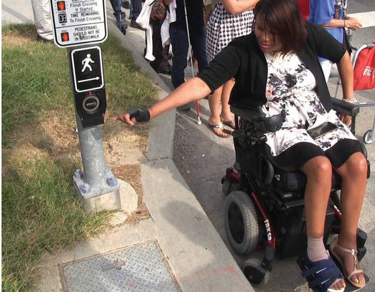
A signal button out of reach makes it nearly impossible for a wheelchair user to cross under the safety of the “walk” light and can be difficult for others to reach, too. Source: planning.org/planning/2018/feb/inclusivemobility/ .
