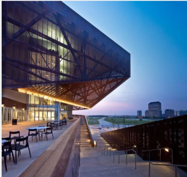
The distinctive Irving Convention Center at Las Colinas features a copper "skin" and a terrace with views of Irving. (Photos courtesy Irving Convention and Visitors Bureau)
