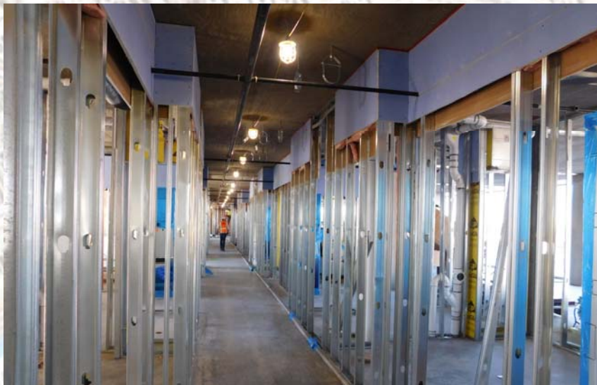
Second Level Hallway and Walls
