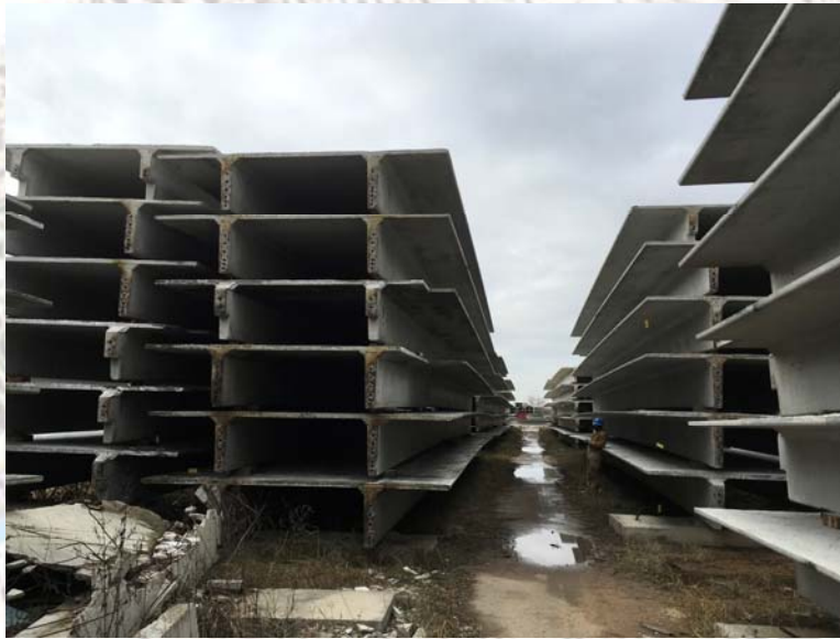
Garage – Pre-Cast T-Beams
