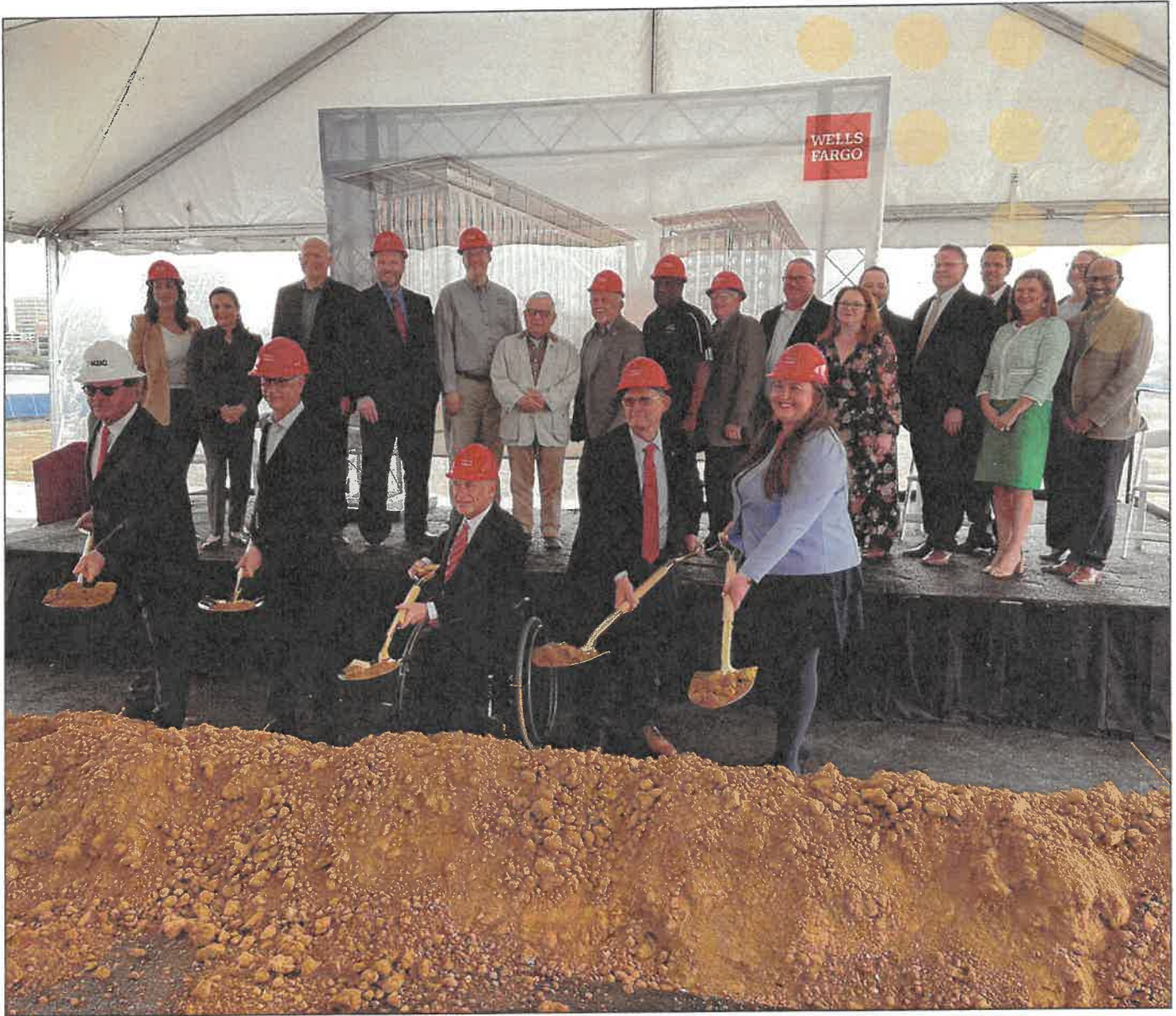
Texas Governor Greg Abbott, Irving Mayor Rick Stopfer, and city and corporate leaders officially broke ground on the new 22-acre Wells Fargo campus near Las Colinas Boulevard and Promenade Parkway, close to the Irving Convention Center, Toyota Music Factory, and DART's Irving Convention Center Station.
