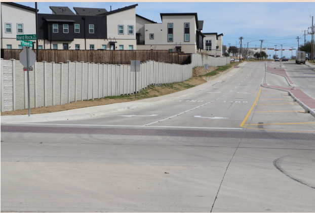
Hard Rock Road and Pioneer Drive (Hard Rock Road from the State Highway 183 Frontage Road to 500 feet north of Conflans Road, and Pioneer Drive from Hard Rock Road to Esters Road) underwent similar enhancements, including roadway pavement and retaining walls adjacent to the lake, at a cost of $9.9 million. Completed Jan. 26, 2024.
