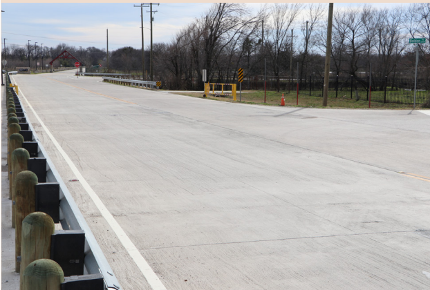
Nursery Road (Delaware Creek Bridge to Hunter Ferrell Road) underwent $7.9 million in improvements, including a hike and bike trail from Oakdale Road to Mountain Creek Preserve Park. Completed Sept. 5, 2023.
