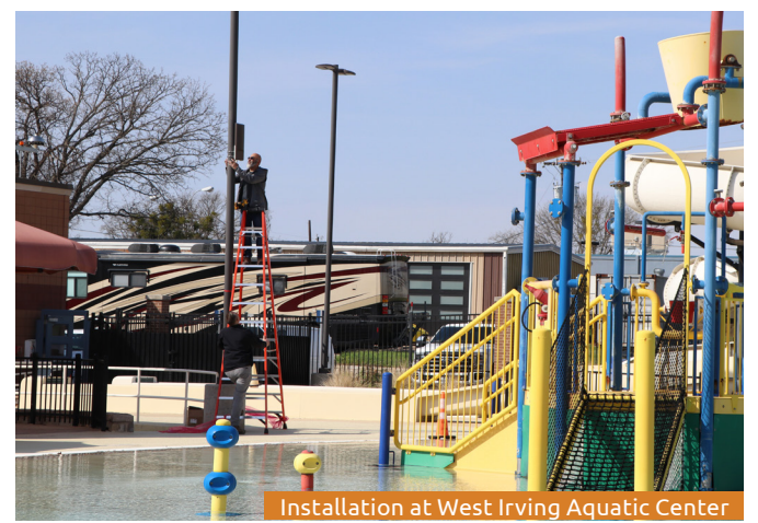
Installation at West Irving Aquatic Center
