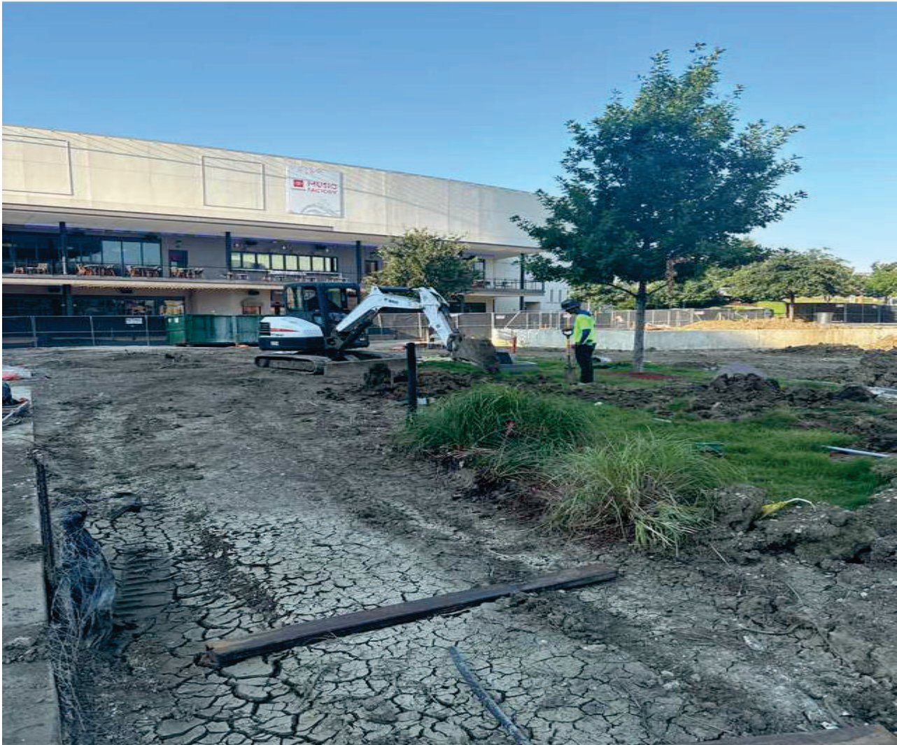
Tying site electrical
