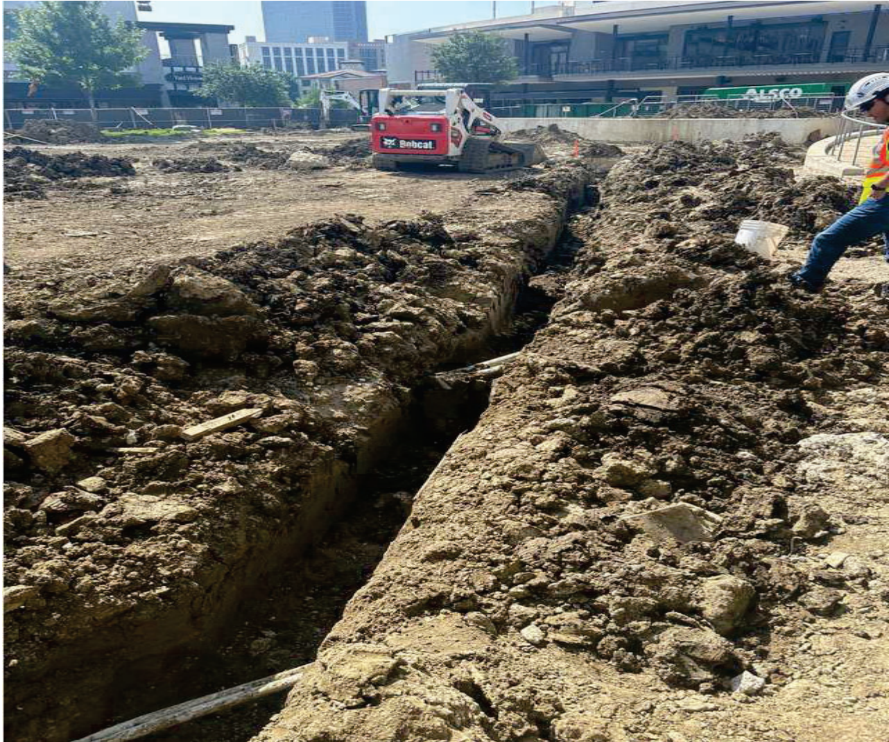
Communication line trenching
