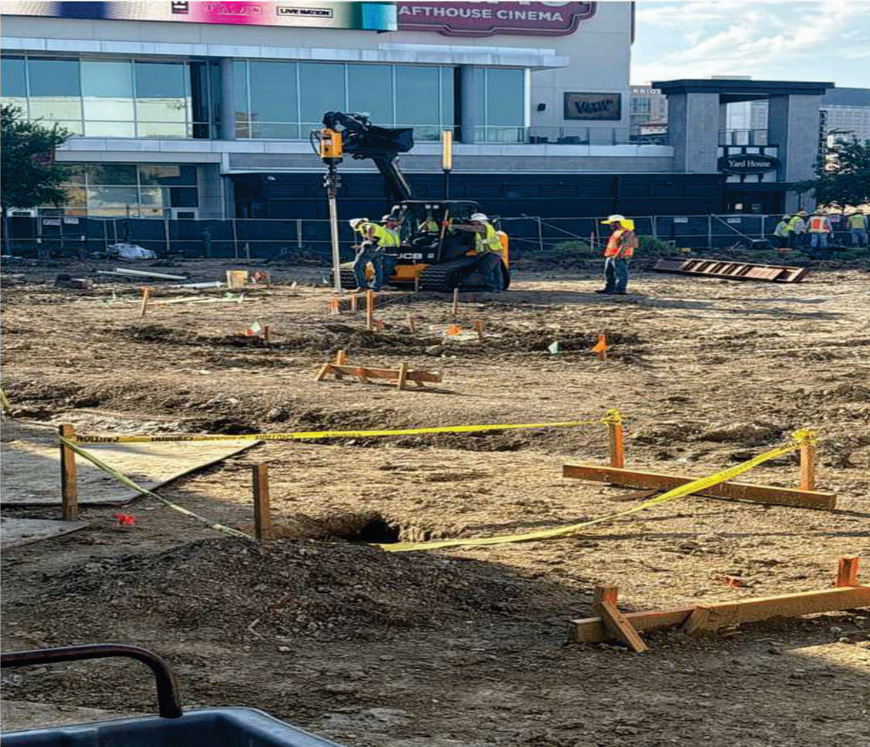
Helical Pile test
