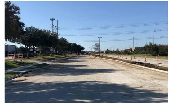
increased pedestrian mobility. In addition, some of the streetlights were relocated and median irrigation was modified and repaired.
