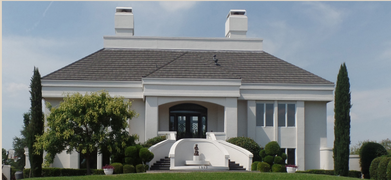
1817 Cottonwood Valley Circle South
