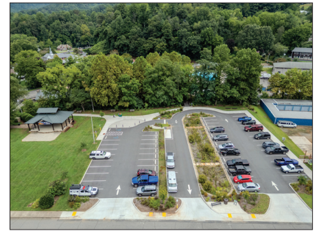
Bridge Park Upgrades FY 23-24 $367,757
