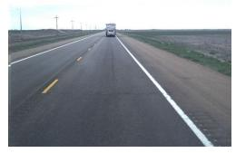
The picture above shows a stretch of U.S. 83 that appears smooth on the pavement surface. However, an inspection of the subsurface (shown below) revealed that the pavement health was in poor condition resulting in having to replace the pavement.
