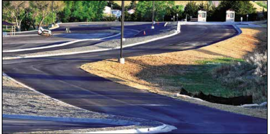
THE RE-DESIGNED ENTRANCE, INCLUDING NEW KIOSKS, AT MARTIN BAY.
