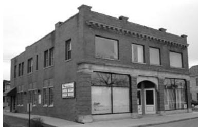
#2 WINBERG BUILDING 1109-1113 – 55th Street (1907) Classical Revival
