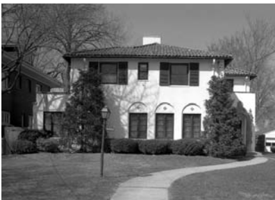
#20 ALEXANDER B. McCALL HOUSE 6334 Third Avenue (1922) Spanish Colonial Revival
