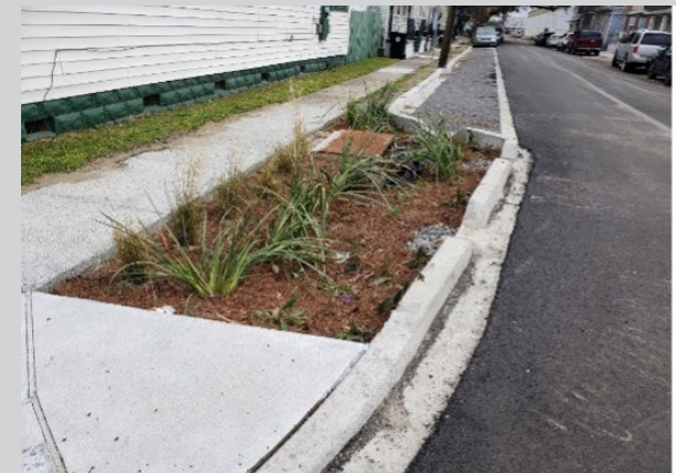
Rain garden and pervious sidewalk and parking system
