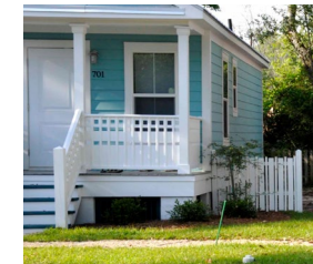
A Pier and beam foundations to raise homes above the path of flooding
