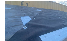
C Secondary water barrier to resist water leaking through the roof
