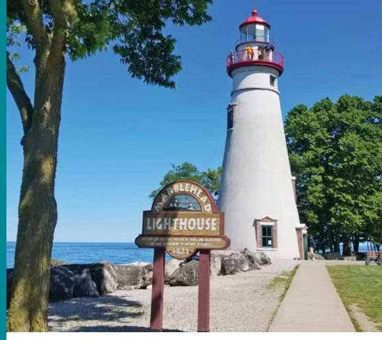
Built of native limestone, the 50-foot tower was constructed by contractor William Kelly as a navigational aid marking the entrance to Sandusky Bay. The base of the tower is 25 feet in diameter, with walls 5 feet thick, narrowing to 12 feet in diameter at the top with 2-foot-thick walls. The original keepers of the lighthouse had to nightly light 13 whale oil lamps, that used metal reflectors to project light across Lake Erie. The oil lamps needed to be refueled every four hours, consuming more
