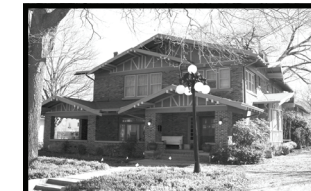
35. 509 Tucker—A circa 1915 Arts & Crafts style home. The exposed rafter tails and low-pitched roof are common to the Arts & Crafts style. Note the beautiful key-hole window located on the west side of the house.
