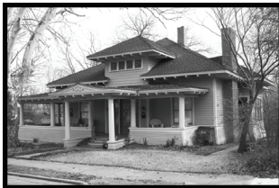
11. 515 W. Hunt—A circa 1915 home designed by J.E. Cooper. The house is a fusion of Classical Revival and Bungalow styles. The owners still have the original architectural drawings
