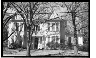
37. 504 Tucker—Built in 1878 by R.M. Board, a local dry goods and clothing storeowner. The house is built on a center hall and originally was two rooms deep. The house is unique in that it has a pressed metal facing in the gables. Note the Palladian window located on the second story above the front door.
