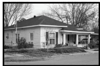
20. 308 N. College—An example of a pyramidal roof vernacular folk house build circa 1915.
