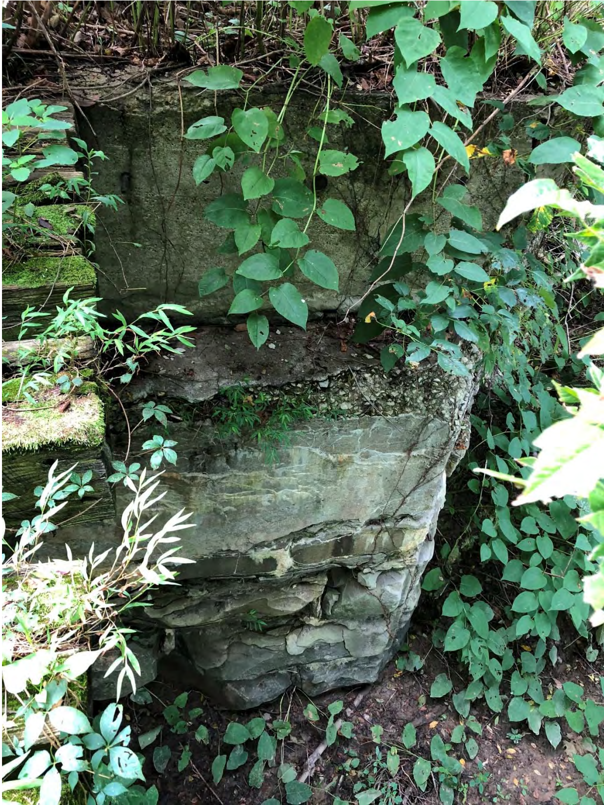
Southeastern Abutment Condition.
