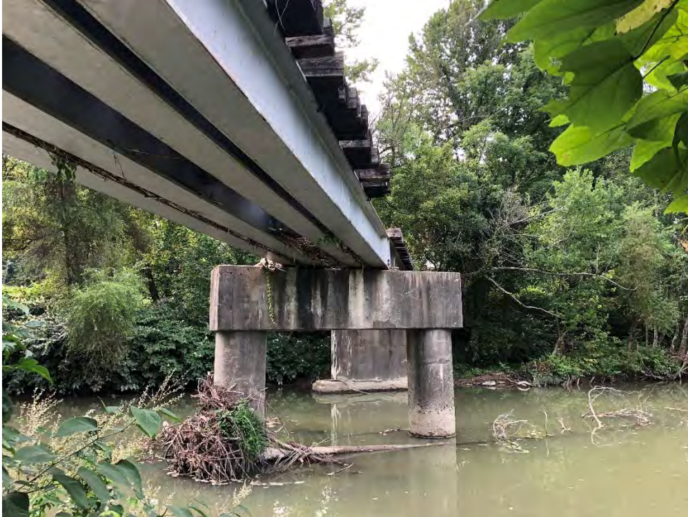
Typical Beam Layout.
