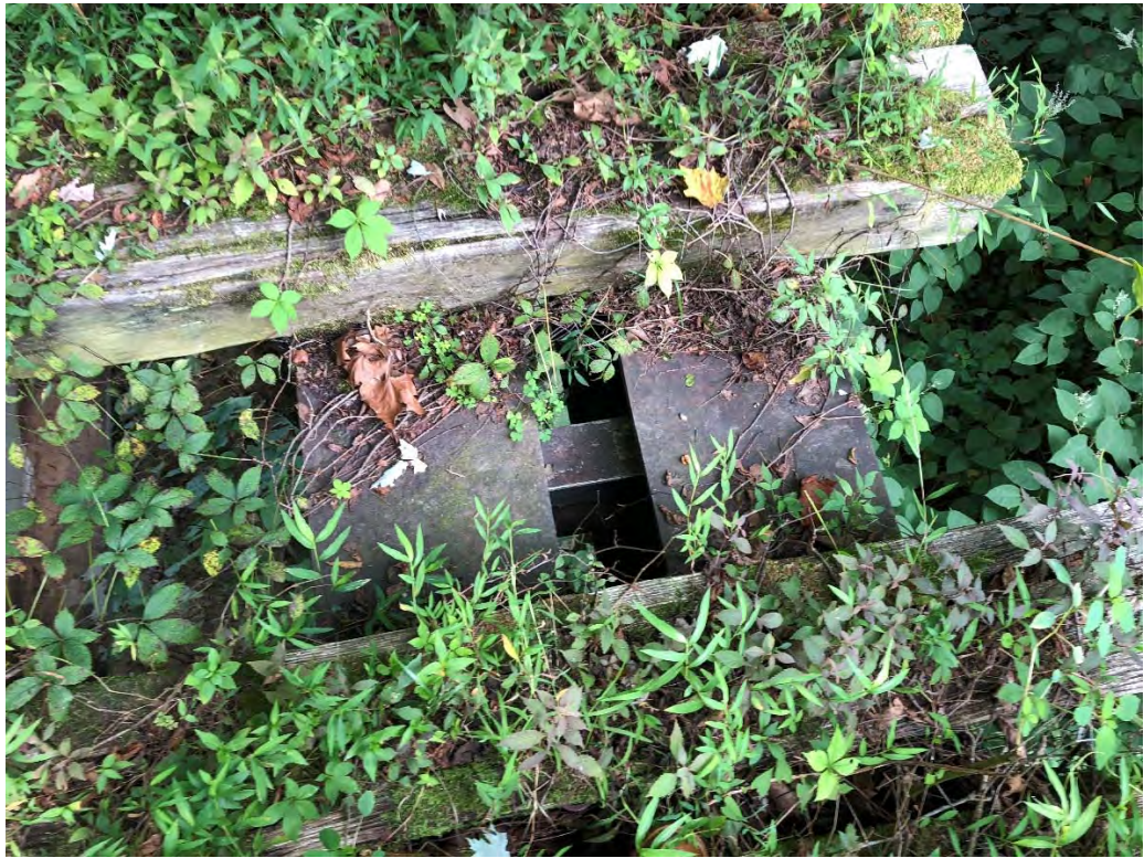
Top of superstructure condition.
