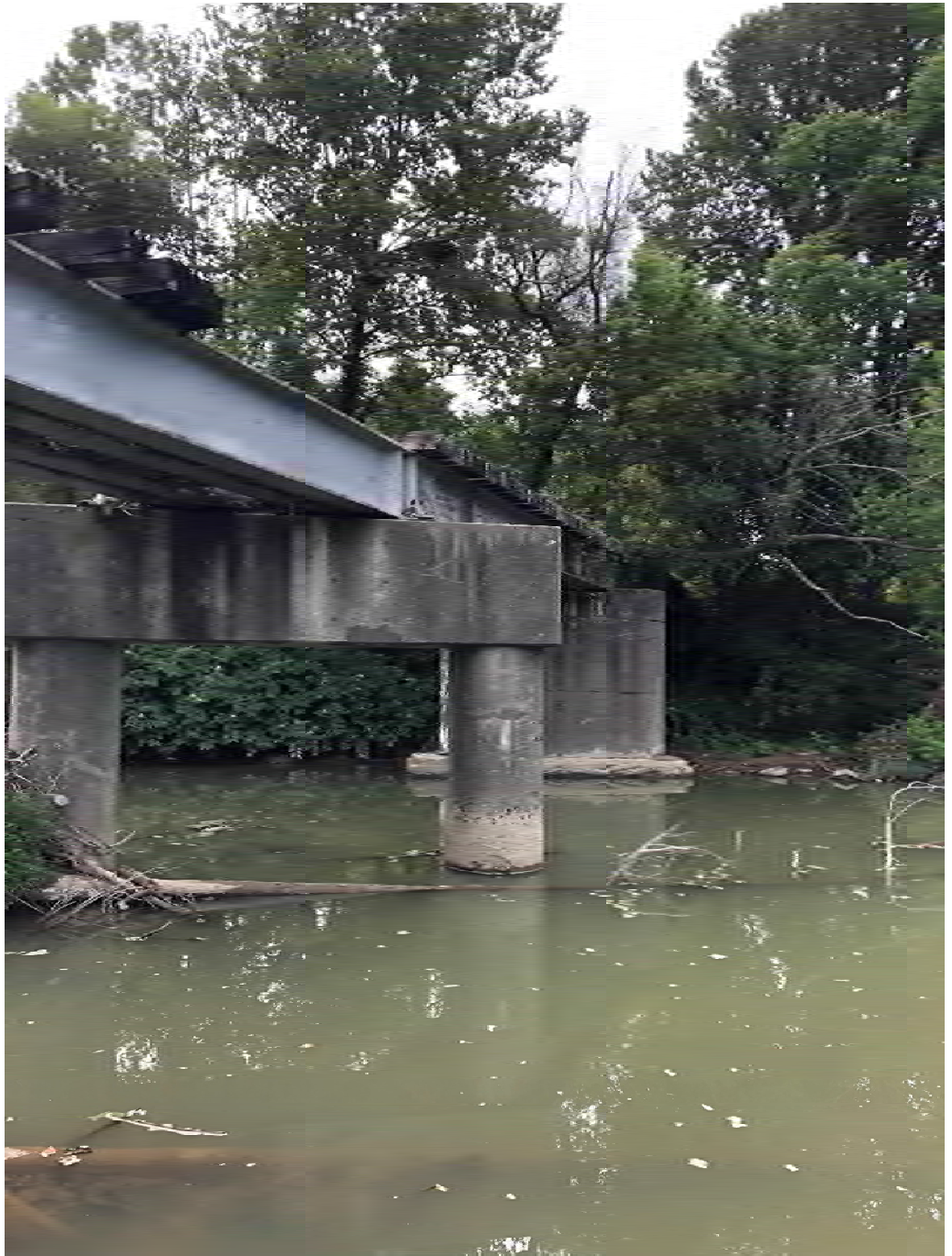
Center Pier with Wall Pier in the distance.
