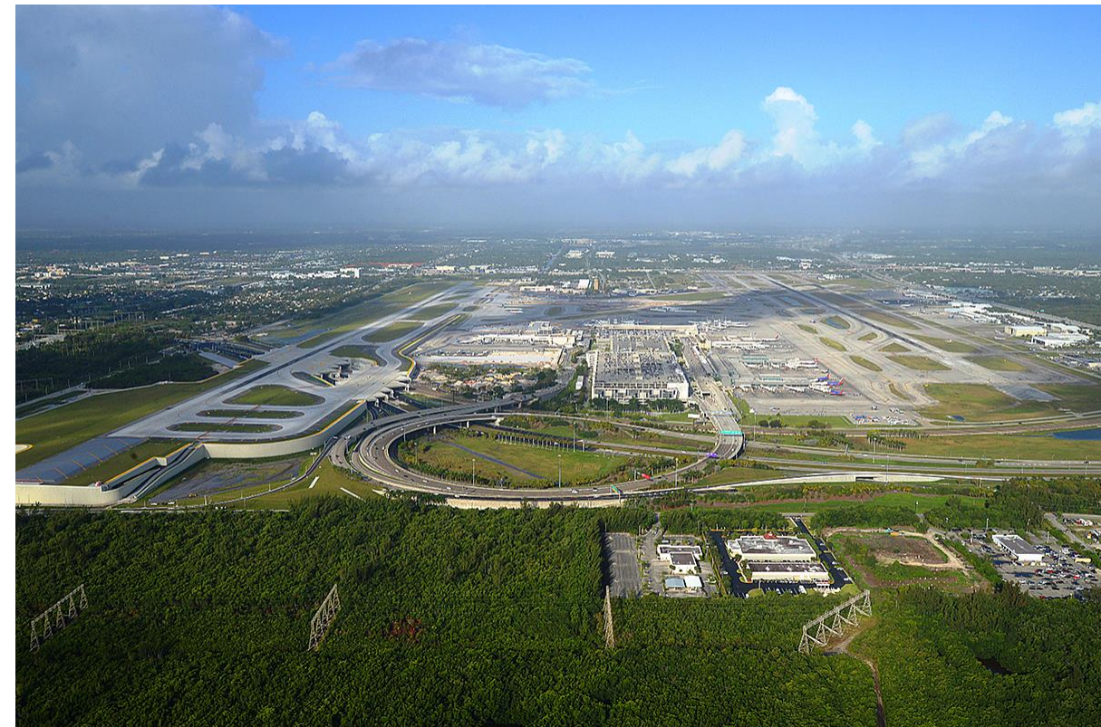
Figure 1.9.9: Aerial View of Fort Lauderdale-Hollywood International Airport (FLL) Source: airwaysmag.com
