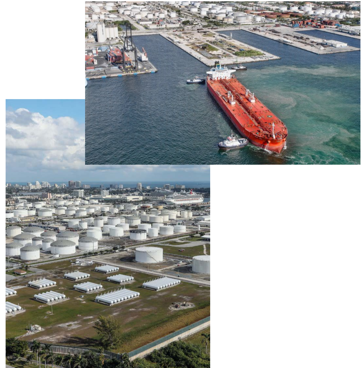
Figure 2.4.12: Port Everglades Liquid Bulk Berths and Storage Facilities Source: Sun Sentinel; Port Everglades
