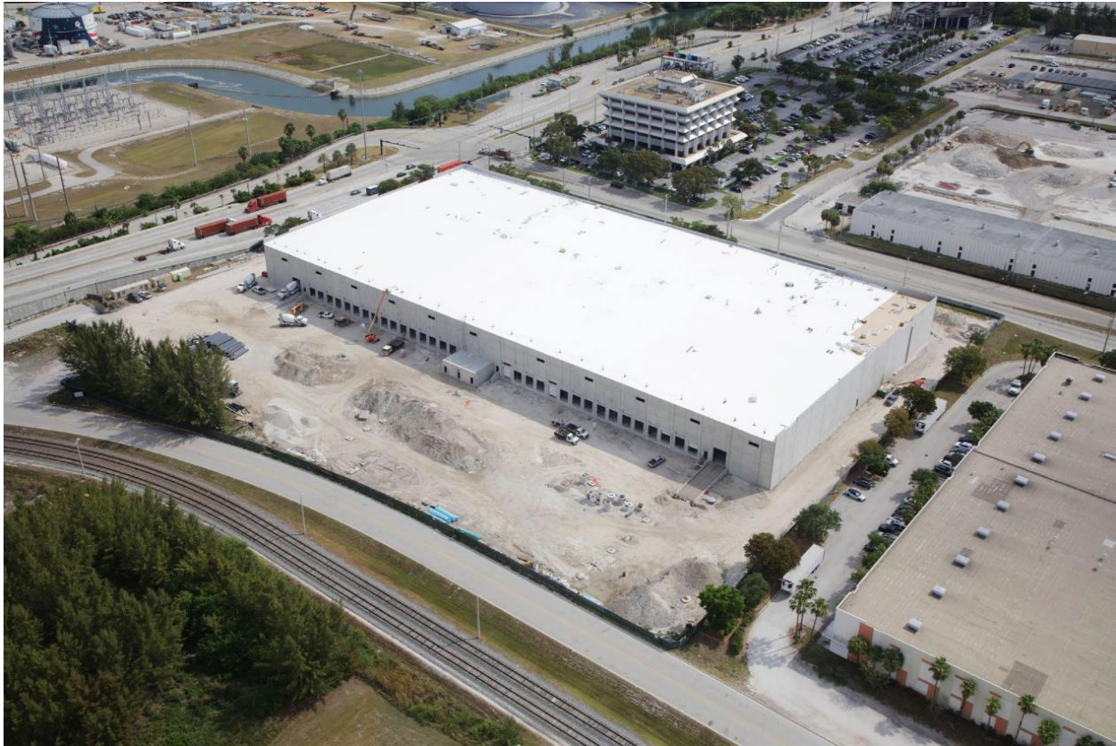
Figure 20. SEAGIS Warehouse Facility
