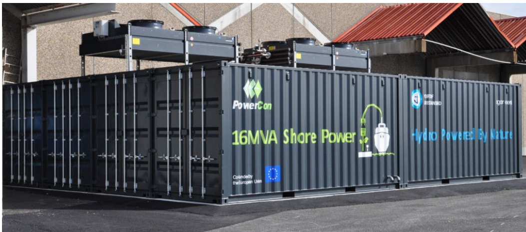
Figure 2-5. Containerized/Contained Shore Power Example
