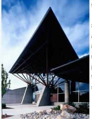
Structural Truss Painting: The trusses that are the architectural focal point of the entrances to the facility need to be cleaned and repainted as part of ongoing maintenance. This project will not only enhance the appearance, but will protect the metal from further degradation. Stallings has been awarded the contract. Work should begin early second quarter, weather dependent.
