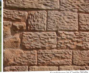
Sandstone in Castle Walls
