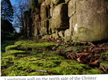
Lapidarium wall on the north side of the cloister
