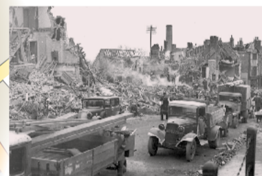
Aftermath of the landmine. Image by Leamington Courier from the Kenilworth Library Collection
