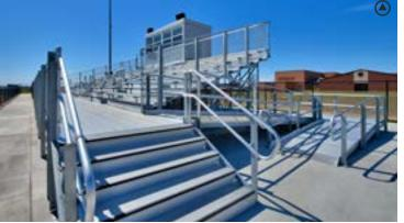
DETAILS The top project featured on the cover is a 57' 10 Row Elevated Angle Frame bleacher that seats 296. Features an 8' x 18' pressbox. Note the galvanized steel framework and aluminum cross braces of the bleacher. Options include the pressbox and ADA ramp. Photos © Todd Brasher
