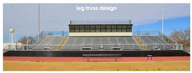
O'Donnell ISD I O'Donnell, TX Leg Truss Design, 12 Rows x 90', Interlock 2000 decking system, 610 Seats, 8' x 48' Sloped front pressbox Features team gold step and black seating risers. Home of Eagle Six-man football and track. Designed, manufactured and installed by Southern Bleacher. Photos: Lane Anderson Photography
