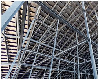
The massive Tarleton State University Memorial Stadium is a testament to our skills. This grandstand offers superior end zone seating. The mitered ends extend around edge of the field, creating a subtle wrap effect. The substructure detail shows the change in angles.
