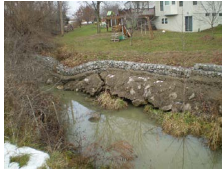
Hard armoring with concrete and gabion baskets on this bank is undercutting, causing more global failure.
