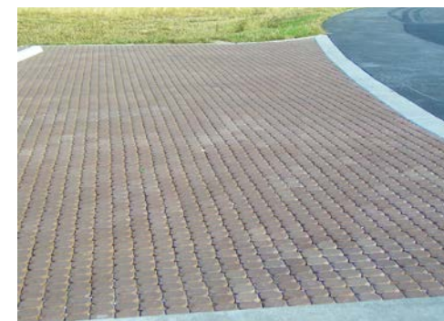
Pervious pavers, Theresa Strunk
