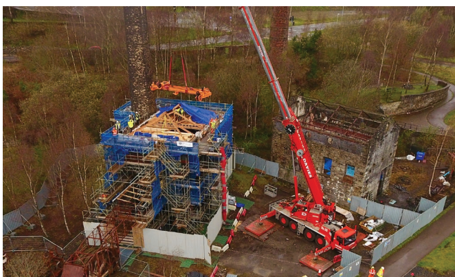
Lowering the restored Gantry Crane into the Musgrave Engine House 2019 © FRIENDS OF HAFOD MORFA COPPERWORKS
