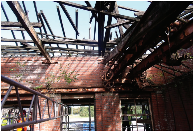
Musgrave engine house and gantry crane 2018, before crane restoration. © SANDY JOHNS
